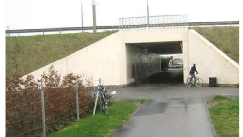
Figure 10.51 Underbridge near Cowley on Oxford Bypass with at-grade approach, wing walls and clear sightlines
